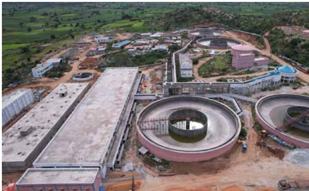
181.45 MLD Capacity WTP at Shivapura, Pavagada MVS (Under construction)
