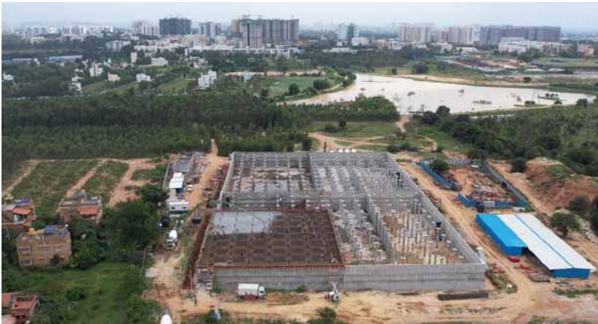
Construction of 48 ML Ground Level Reservoir at Doddakanahalli under progress
