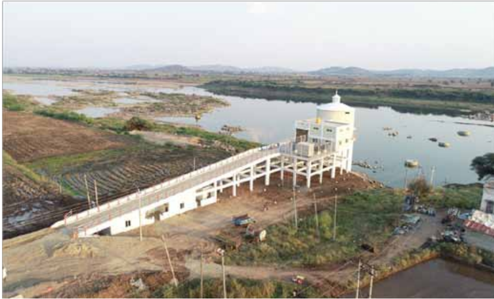
Head Works under 2 nd Stage WSS to Shorapur Town & 3 Enroute Villages with Krishna River as Source
